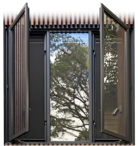
After-market or retro-fit systems often look like an obvious addition to the existing window. Rylock Acoustic Series products integrate both primary & secondary window elements inside the one reveal box, making for an attractive solution for noise attentuation
