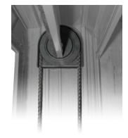
Pre-stretched, engineered rope runs through the counter balance pulleys.
